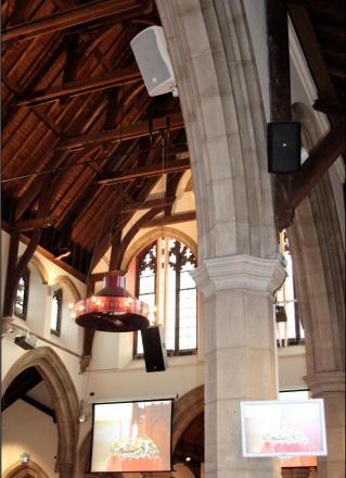
Picture showing the central flown Xi2123a speaker, relay ZX3 and ZX1i speakers and projection system
