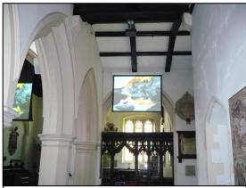
One of the two side aisle screens featuring 3000 lumen Eiki projectors and remotely operated motorised screens
