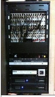
Vestry rack including EV Netmax processor, audio & loop amplifiers and patching system
